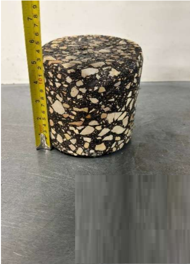
BH17 - Eastbound Lane
