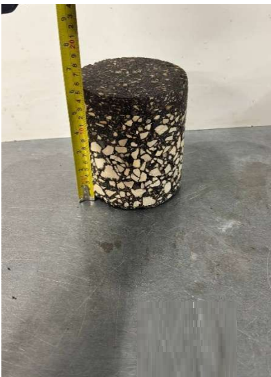
BH14 - Westbound Lane
